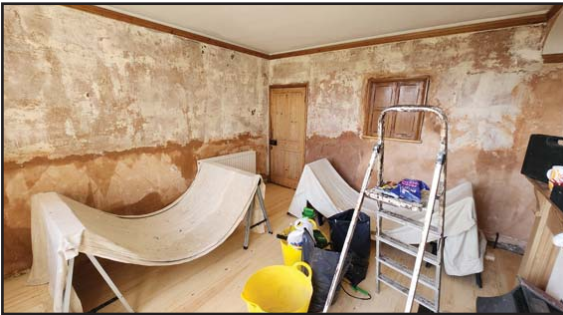
Work in progress on no. 8
